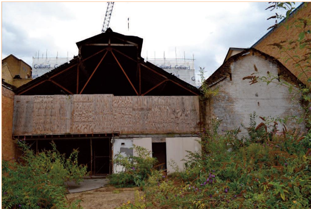
Figure 8: Site A and the rear of the partly demolished buildings
